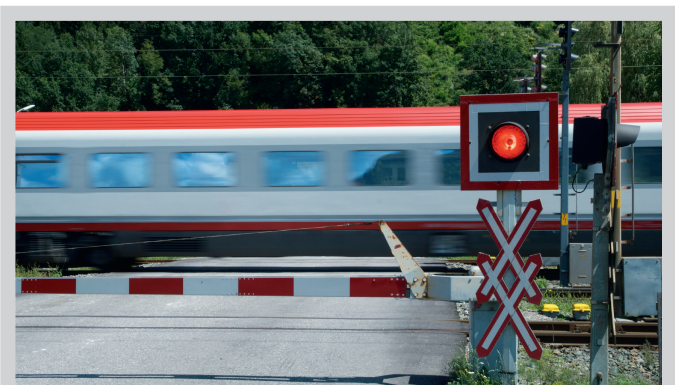
Figure 2: Trend towards wheel detection and axle counting to control level crossing protection systems
