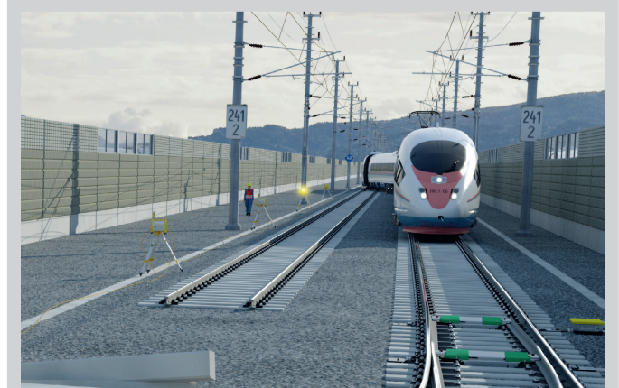
Figure 4: Automatic warning systems are controlled by wheel detection systems
